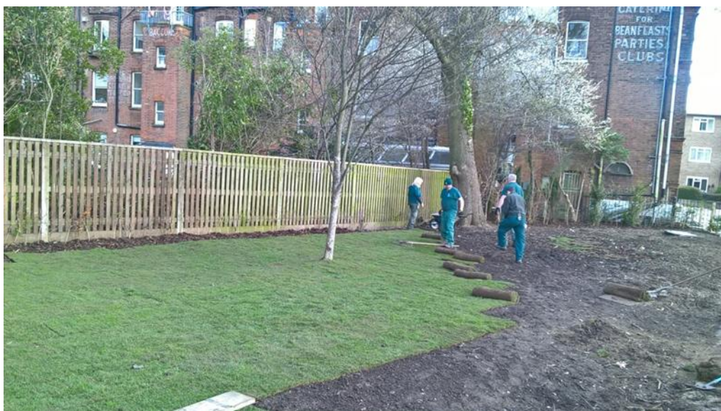
Figure 5: Swain's Lane landscaping works in progress
