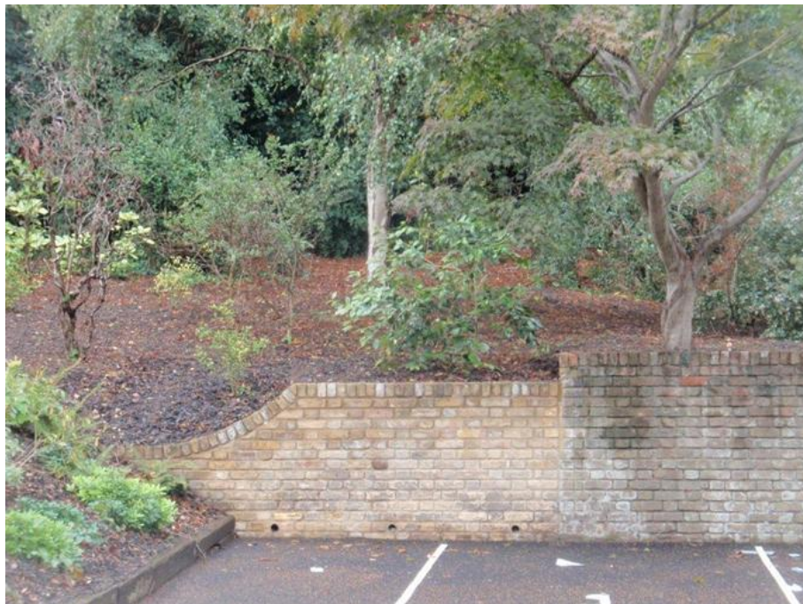
Figure 4: Disabled car park re-landscaping
