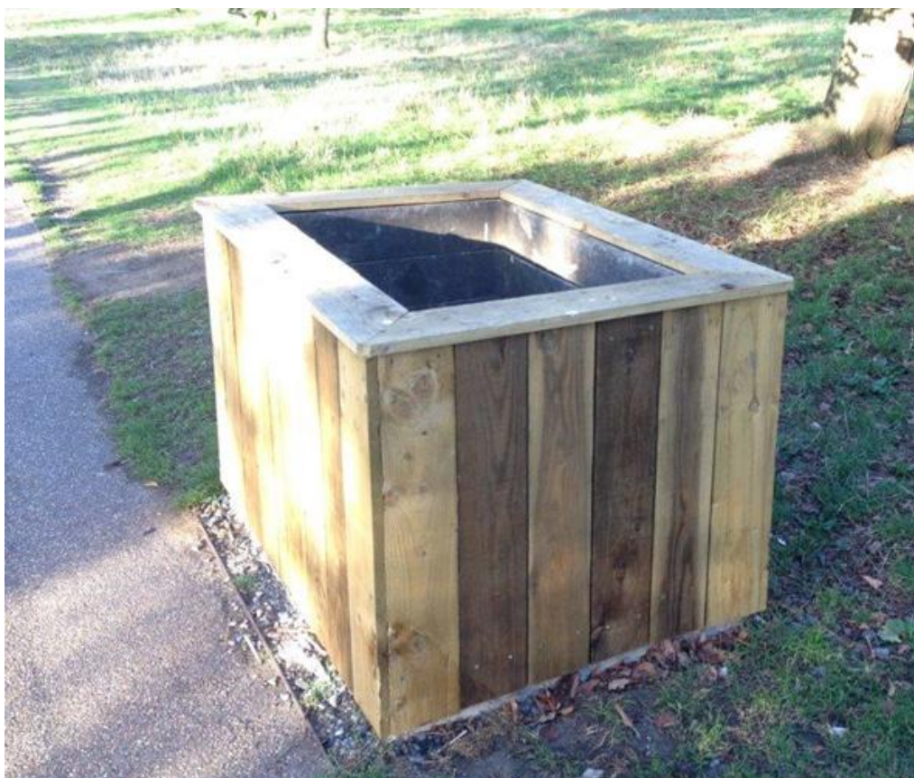
Figure 6: Bin with new wooden cladding
